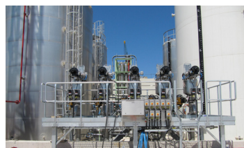
Advanced filter System w/forced ventilation and emergency shutdown
